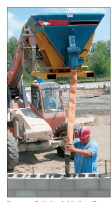
Masons can effortlessly swivel the Groutzilla hopper and move the discharge hose along the wall, filling as they go to cover a substantial length of wall before the unit needs repositioning.
